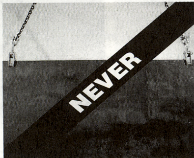
Photograph G (Typical)
